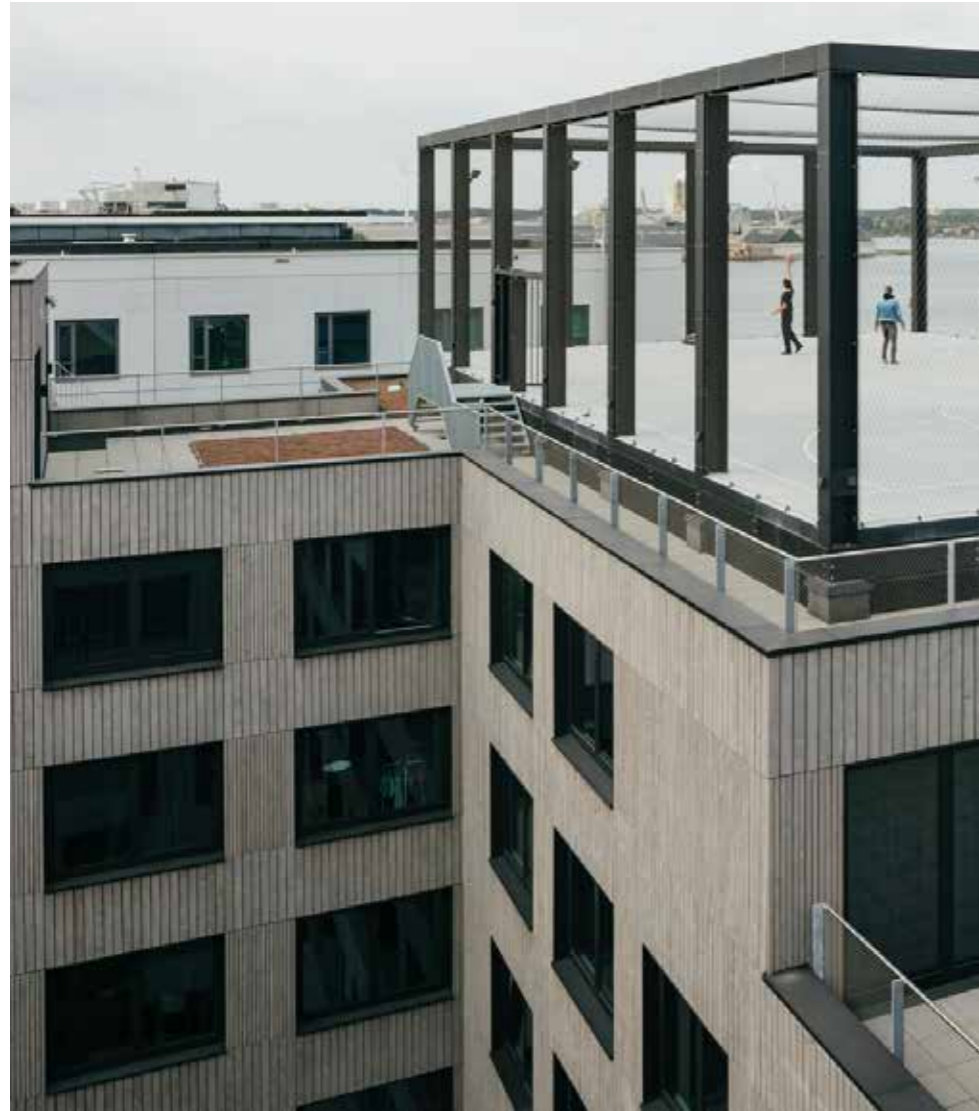
Student Experience Minervahaven / VURB Architects
