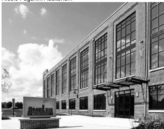
Ambler Boiler House
