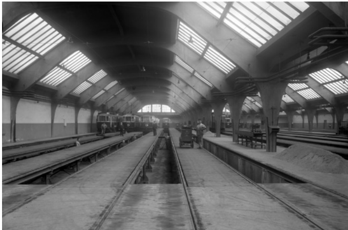
interior of the depot hall with carriage inspection troughs
