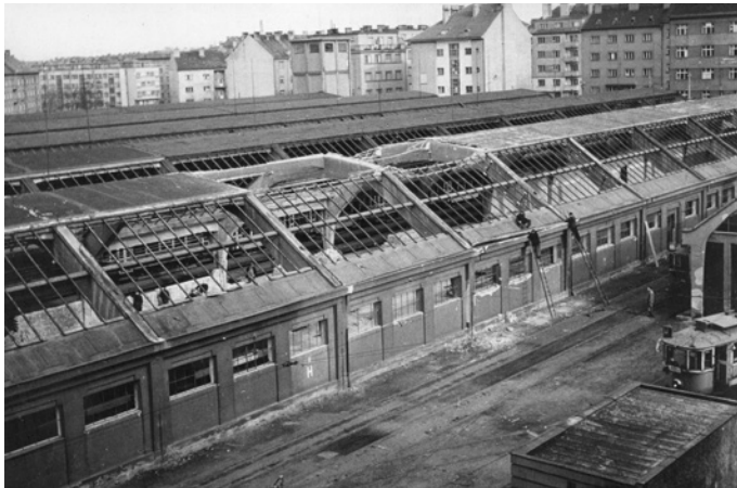
collapsed roof structure after an impact of a bombshell in February 1945
