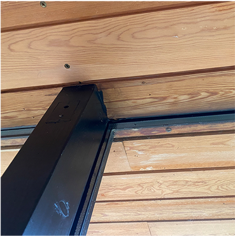
Close up photo of glazing detail - no frame - structure is the frame
